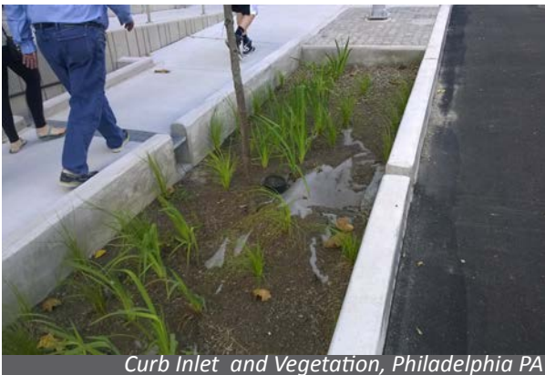
Vegetated Stormwater Inlet, Philadelphia PA
