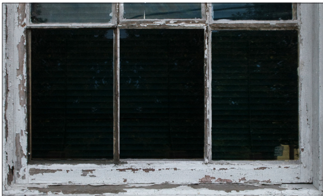
Often, the deterioration of wood windows first occurs at the sill. Peeling paint can allow moisture to enter wood and cause rot. Regular repainting is recommended to provide a protective layer against moisture.
