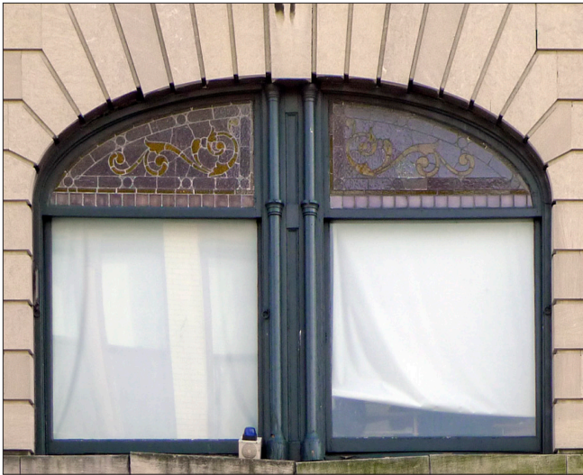
Historic windows were often seen as a design feature. This example includes a decorative wood surround and stained glass in the transom above an operable casement sash.
