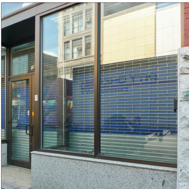
Security grilles should be open weave and located at the interior behind storefront display areas and entrances whenever possible.
