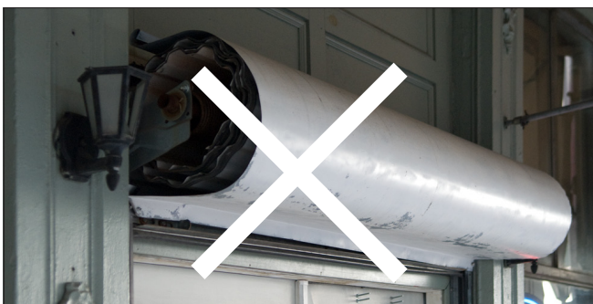
Exterior security grille housings are not permitted.
