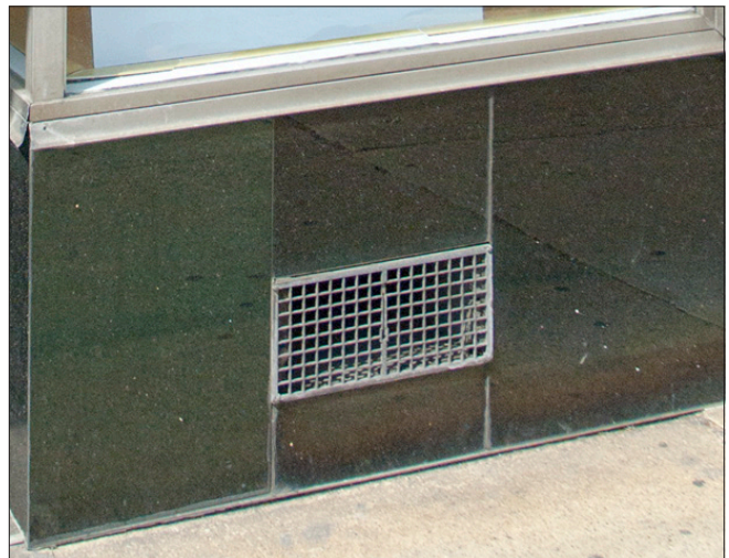
This polished granite apron provides the base for the storefront window and includes a metal vent.
