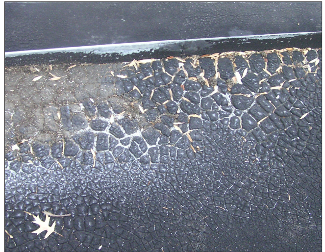
The alligatorated roof surface indicates deterioration and is in need for replacement.
