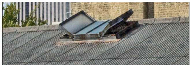
Some skylights were historically located in warehouse and commercial buildings, providing natural interior light and ventilation. The visibility of new skylights should be minimized.
