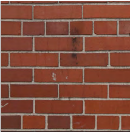
20th Century Brick - A hard, dense, fired-clay, regularly shaped building component; sometimes with a glazed surface; used primarily in walls, piers, foundations and exterior pavers.
