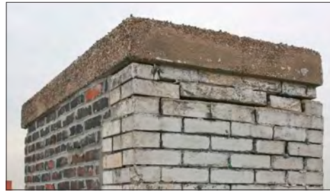
Roof features, such as this chimney, need regular maintenance, particularly to prevent storm water from entering a building.
