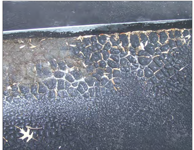
The alligatored roof surface indicates deterioration and is in need for replacement.
