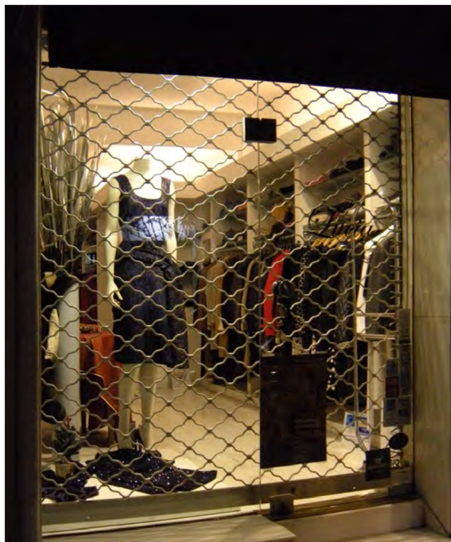
Interior open-weave security grilles provide protection while allowing the merchandise to be visible when the store is closed.
