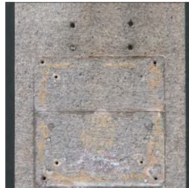
Numerous holes have been drilled into the face of this granite pier and several previous fasteners remain.
