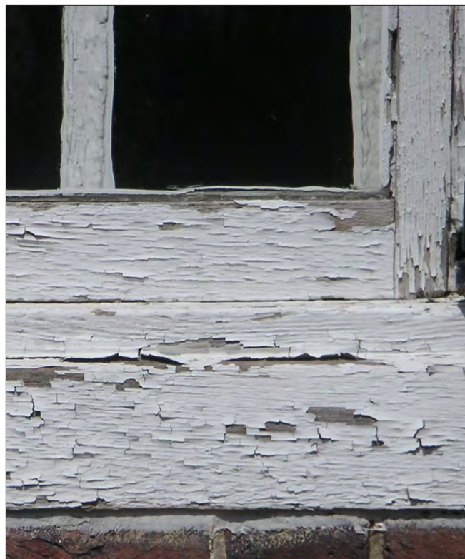
The window sill and jamb have peeling paint and some checking or splitting. Removal of the loose paint will allow the wood to be inspected for signs of rot.
