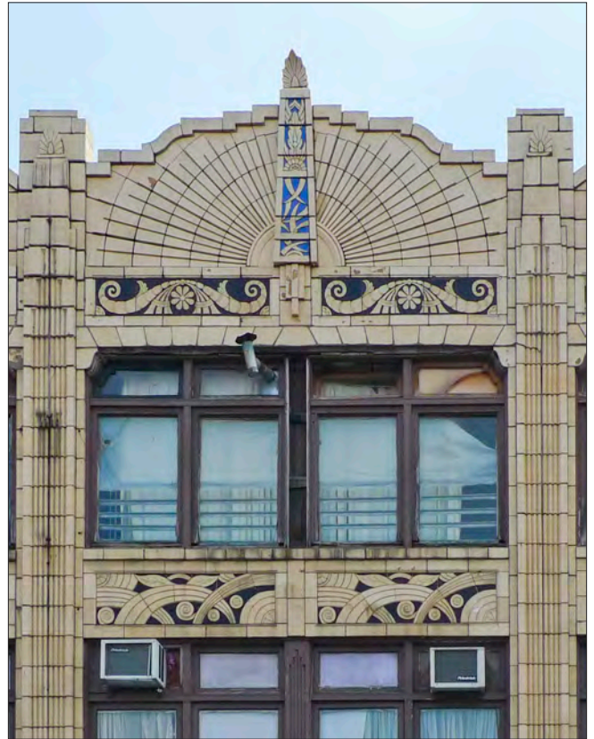
The way terra cotta is manufactured allows for a variety of shapes, forms, and colors. This example celebrates the Art Deco style.
