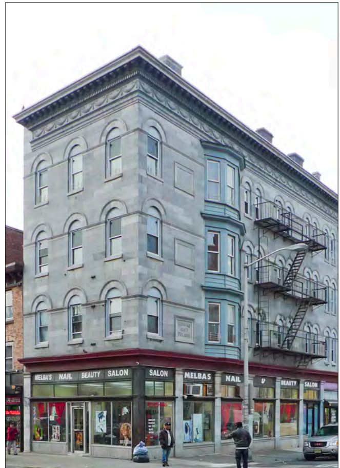
This four-story building retains the three vertically stacked zones, typical of commercial buildings, namely the ornamental cornice at the top of the building, punched windows on the upper floors, and the storefront with large display windows at the ground floor.
