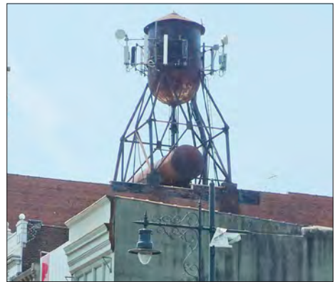
Water towers were a common rooftop feature on commercial buildings in Paterson. They provided water for occupants and were used for fire fighting.
