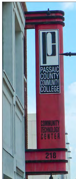
Larger scale projecting signs that are mounted to the building at the top and bottom such as this example are sometimes referred to as blade signs.
