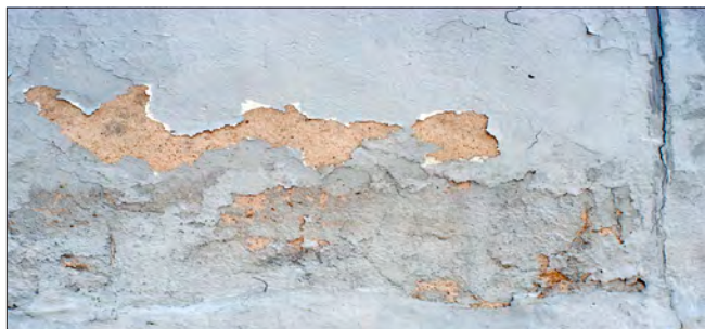
When painting stucco, it is recommended that a breathable masonry paint be used and that loose or flaking paint be removed prior to repainting.
