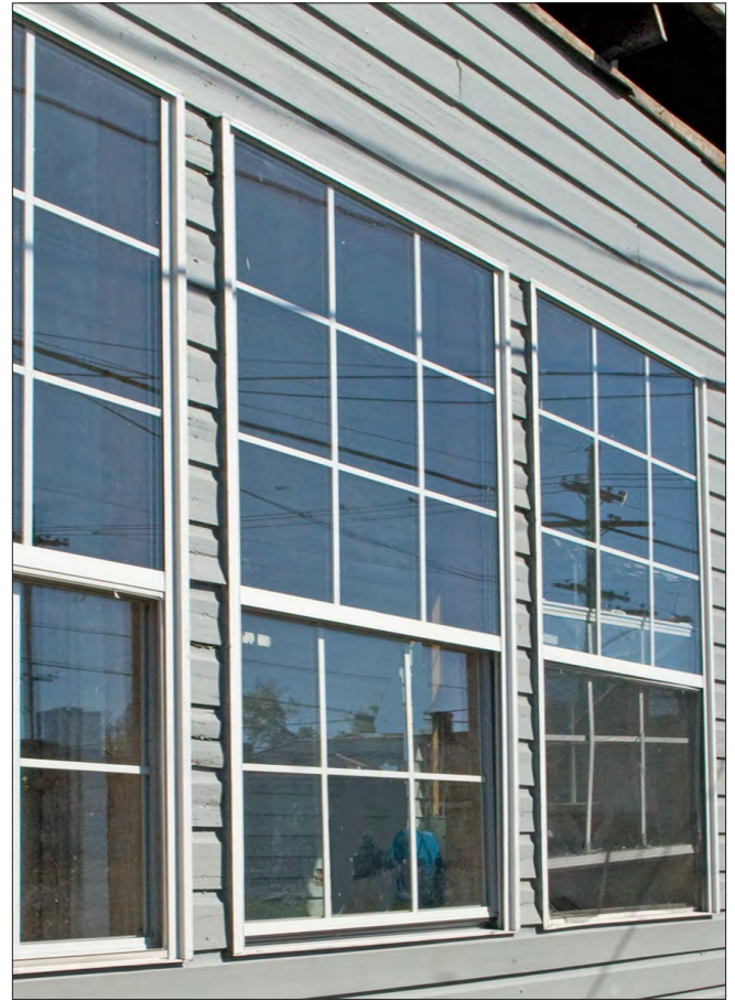
These low-quality 9-over-6 vinyl replacement windows have applied muntins, are mounted flush against the outside wall and lack the depth of traditional windows. They do not have sills to direct water away from the building wall below or exterior trim. The window to the right is wracked, or twisted in its opening and it does not appear it will close properly. They are not appropriate for historic buildings.
