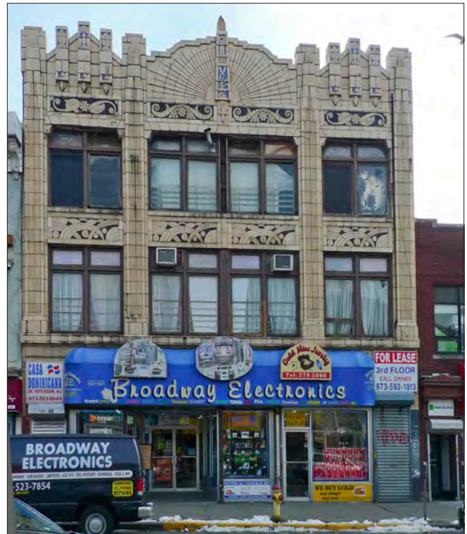
Art Deco: This early 20th century structure displays the typical Deco stylings including geometric and floral terra cotta details as well as fluted pilasters between window groupings.
