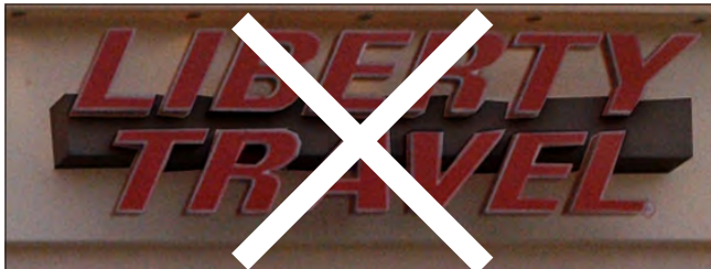
Exposed raceways for channel letter signage should be painted to match the adjacent wall surface.
