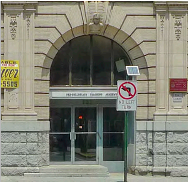
The two steps at the right side of the opening were cut-down to allow wheel chair access from the sidewalk.
