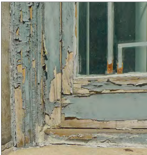
Regular repainting of exterior wood elements, such as windows, can protect them from wood rot and costly replacement.
