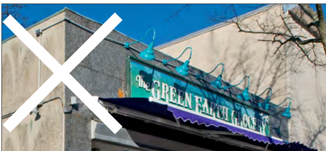
Conduits should be concealed and not mounted to the face of the building. The number of lamps should be reduced to provide enough light for the signs to be read.
