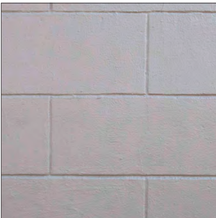
Scored Stucco - Smooth finish with scoring to simulate stone joints.
