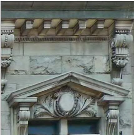
Limestone - A sedimentary rock; used for building walls, window sills and lintels, ornamental stone, sculpture and for producing lime.
