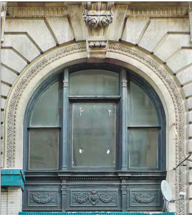
The three cast bronze spandrel panels have a cast swag pattern and separate the arched window from the doors below.
