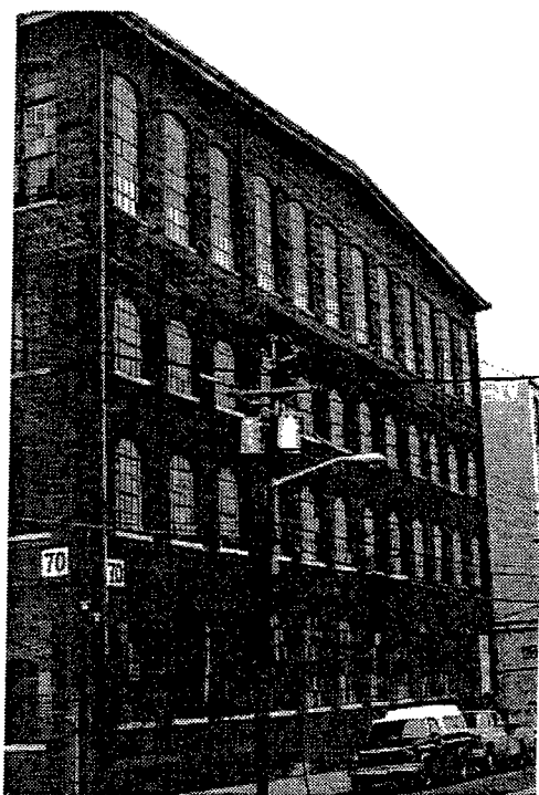
The Dolphin Jute Mill main building, built in 1880. The fourth floor was added later.
