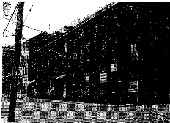
The manner in which the original window openings were bricked up at the Rogers Locomotive Millwright Shop has completely changed the character of the building.
