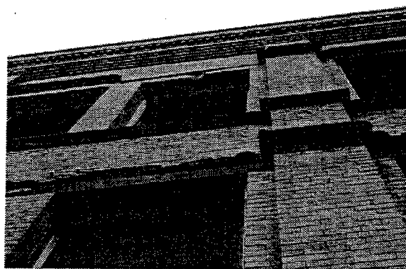
Brownstone deterioration at window surrounds and belt courses of the Cooke Locomotive Company Office Building.
