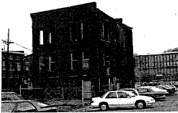
When restoration of the Cooke Locomotive Company Office Building takes place, the cornice on the north wall of the building should be replaced, preferably restored to its original configuration with brick. A substitute material may also be acceptable.
