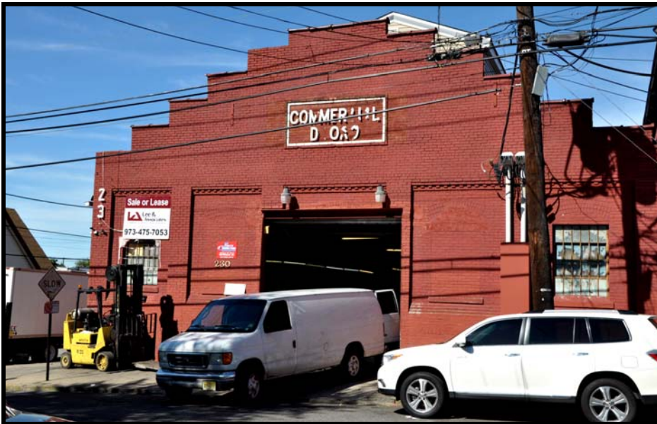
AIRCRAFT 3: View looking west of the 16th St. entrance to one-half story machine shop building that occupies the length of the block along 8th Ave. Corner of 8th Ave is at left frame.
