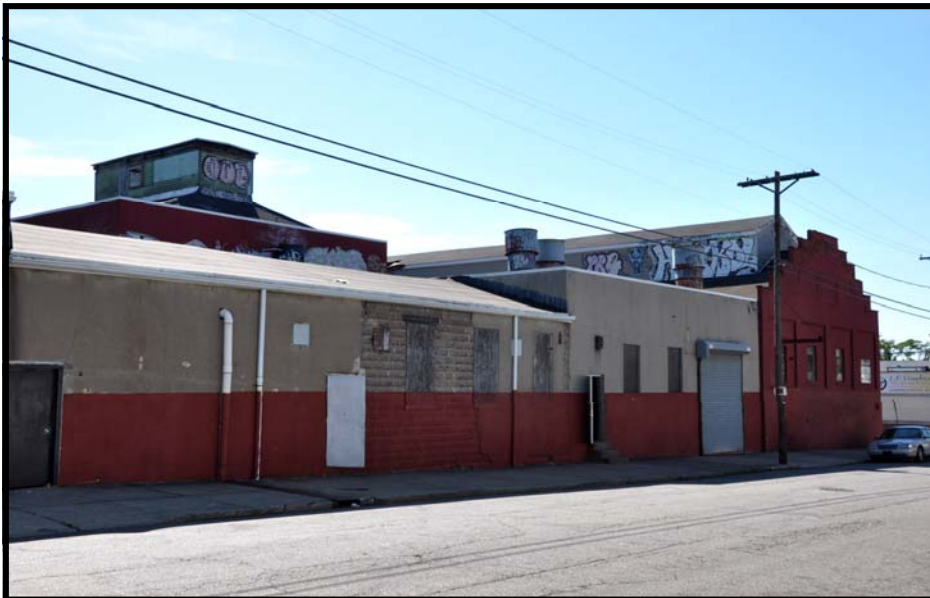
AIRCRAFT 7: Oblique overview of complex along East 15th St. looking south. The recently refinished buildings in foreground may have been the paint shops.
