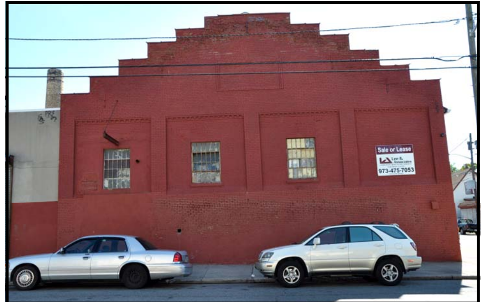
AIRCRAFT 8: View of rear elevation (west) of the one-half story machine shop building that occupies the length of the block along 8th Ave.
