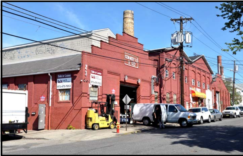
AIRCRAFT 1: Oblique overview of complex facades along East 16th St. looking north from corner of Eight Ave. and East 16th St..
