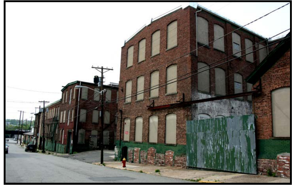
ASHLEY 4: oblique overview along Warren St., looking NW.
