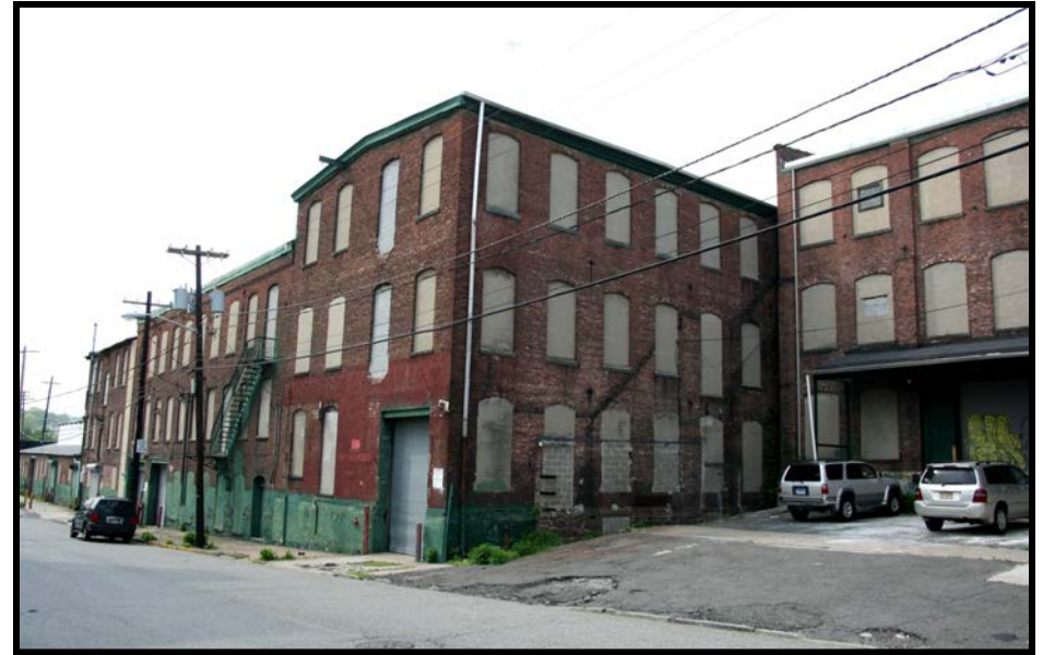
ASHLEY 2: Oblique overview looking NW along Warren St. showing east and south elevations of mills.
