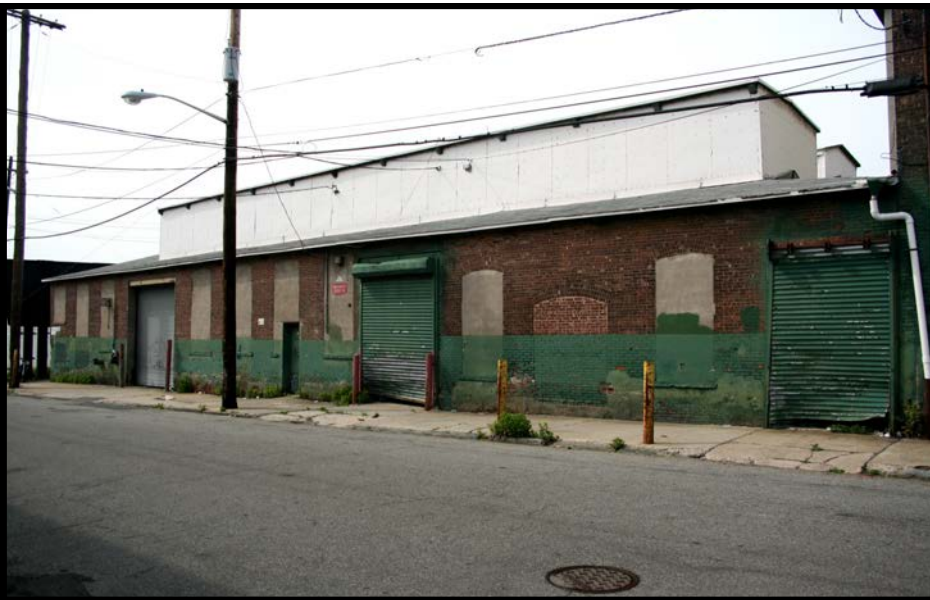
ASHLEY 7: Oblique overview looking NW from across Warren St. showing a Dye House at corner of Warren and River St.
