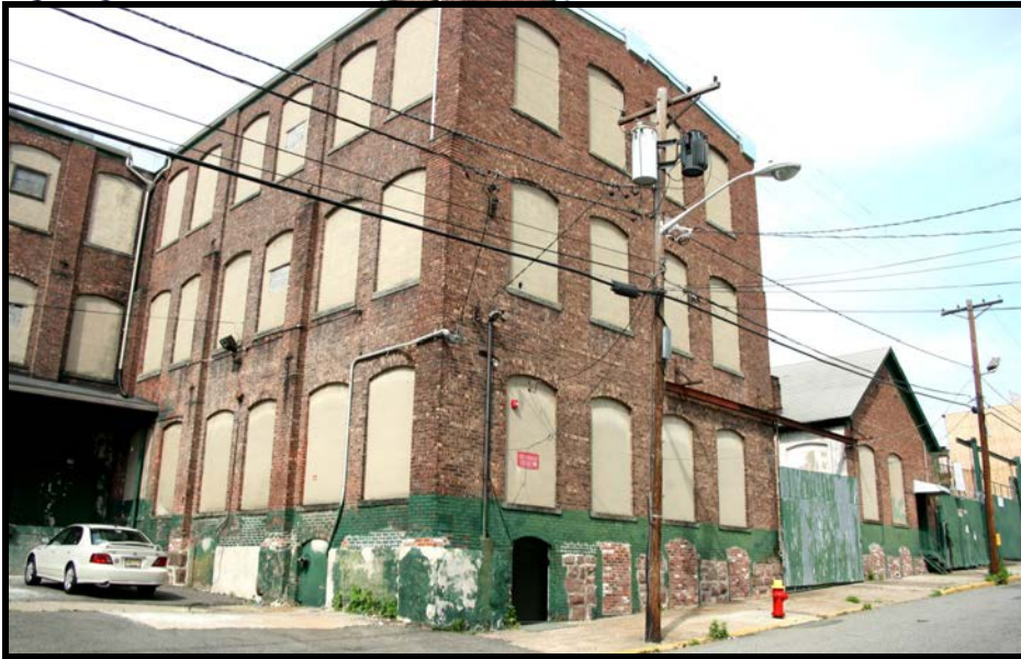
ASHLEY 3: Oblique overview looking NE along Warren St. showing W and S elevations.
