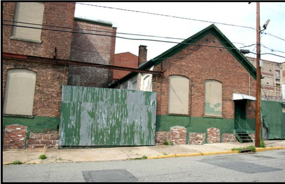
ASHLEY 5: View looking N from across Warren St. at east end of site.
