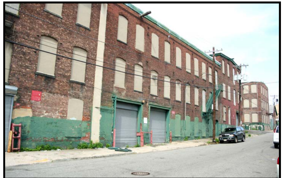
ASHLEY 8: Oblique overview looking NE along Warren St. showing south facades of mills.
