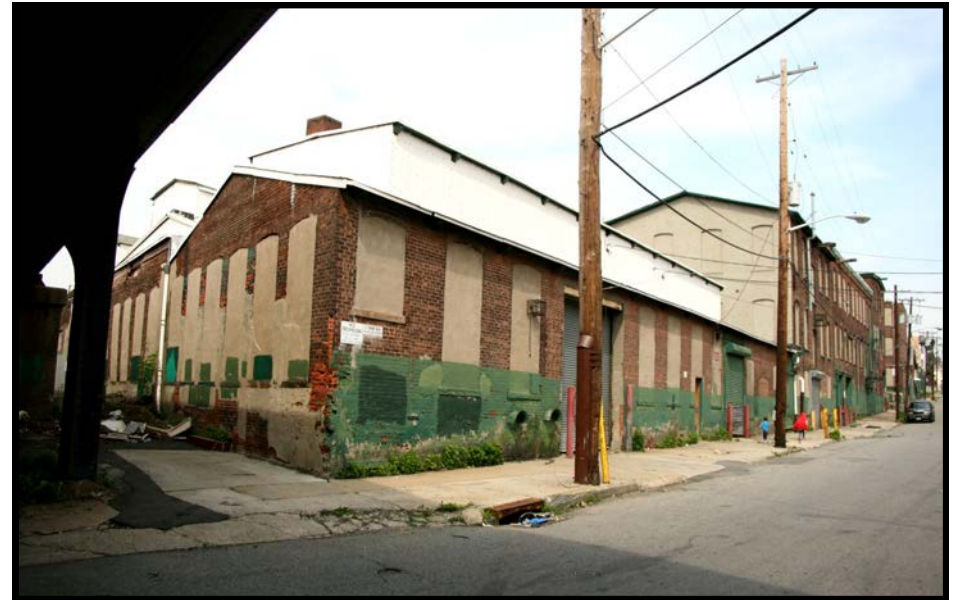
ASHLEY 6: Oblique overview looking along Warren St. from under trestle at corner of Warren and River St..
