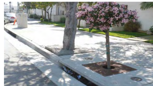
Stormwater Bioretention Inlet Image from Filtera website
