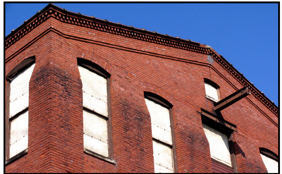
HALL 4: close up view of 1910s building east gable end, looking NW. Details of interest are clearly shown: meticulous brick corbelling and running course work of the closed eaves, the terra cotta coping, and the gradual-stepped buttressed pilasters.
