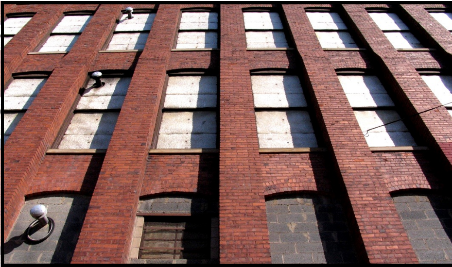
HALL 19: detail view of South side of 1910s building, looking N from Harrison St., showing consistent, reversible modifications to window openings (fenestration).
