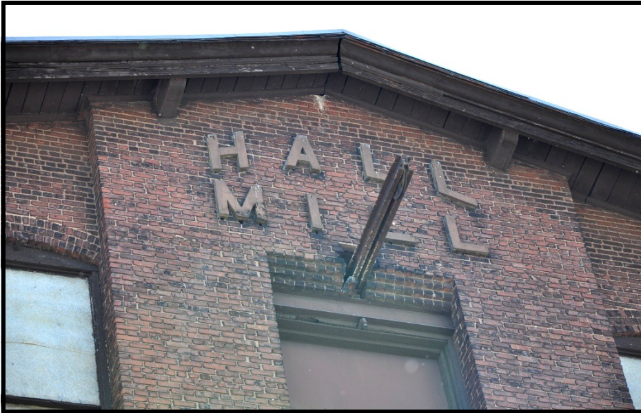
HALL 11: close up view of West gable end of the 1899 mill building addition, looking E from Straight St. showing the Hal Mill name in sandstone lettering. The integrity of the open eaves and cornice moldings emphasizes the historic character of the mill addition.
