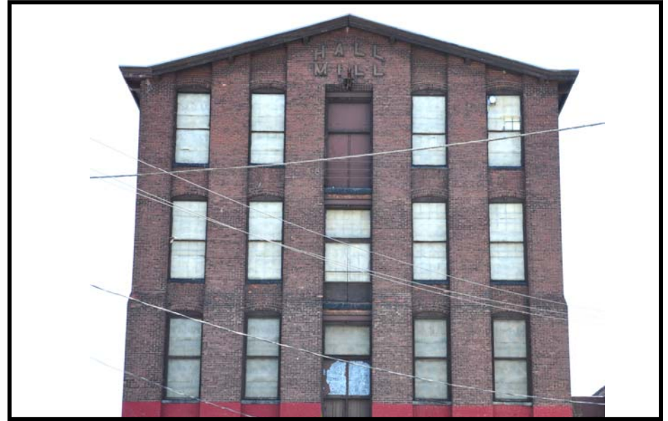
HALL 10: detail view of West gable end of the 1899 mill building, looking E from Straight St. The integrity of this façade is clear, including the covered original windows
