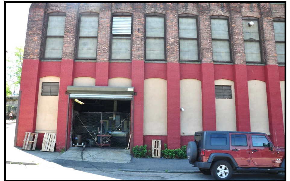
HALL 8: detail view of 1899 building, looking S from Fulton St., showing a double bay entrance modification made to accommodate a machine shop tenant.
