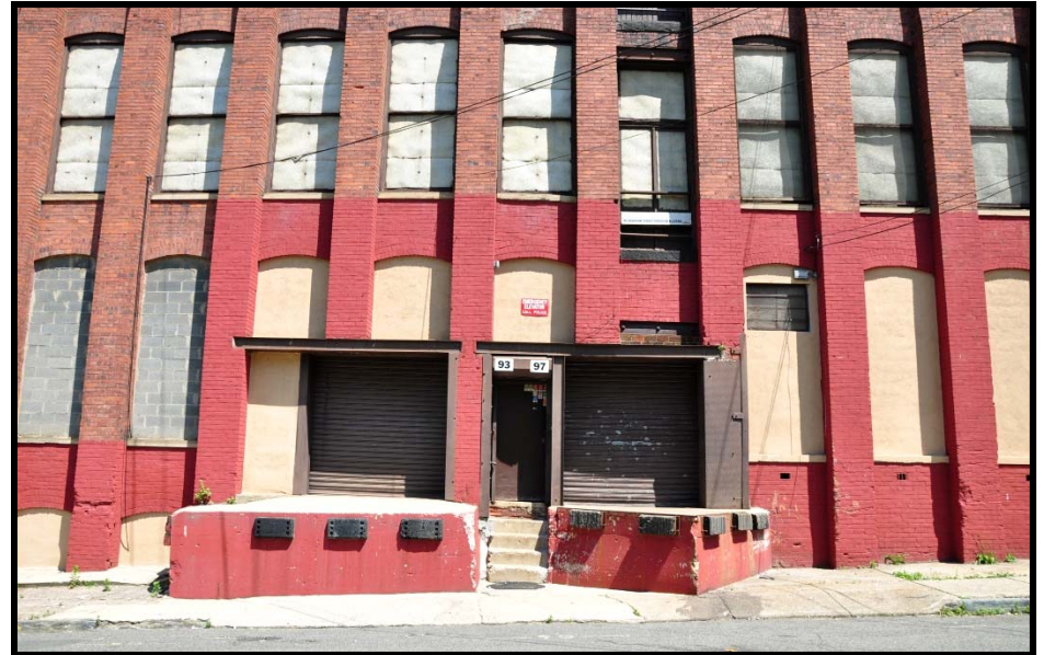
HALL 16: detail view of South side of 1910s building, looking N from Harrison St., showing several loading dock and entrance modifications made to accommodate tenant reuse.
