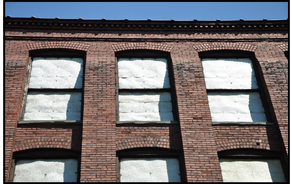
HALL 18: detail view of South side of 1910s building, looking N from Harrison St., showing brick dentils, stringcourse detailing, and use of terra cotta coping. Segmental arched windows may be extant behind the white covering material. Integrity is clear.
