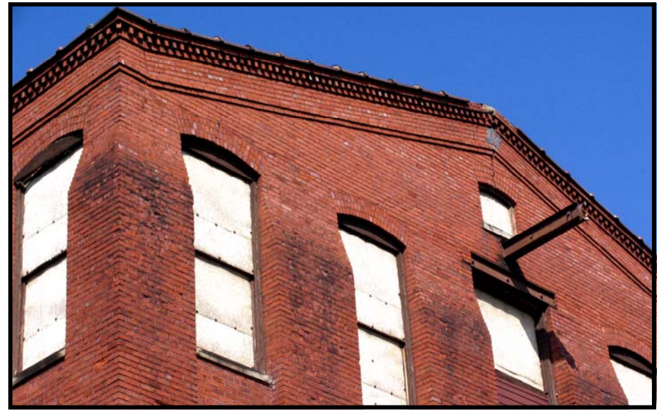
HALL 4: close up view of 1910s building east gable end, looking NW. Details of interest are clearly shown: meticulous brick corbelling and running course work of the closed eaves, the terra cotta coping, and the gradual-stepped buttressed pilasters.
