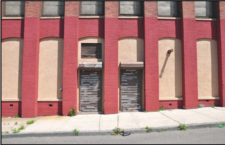
HALL 17: detail view of South side of 1910s building, looking N from Harrison St., showing additional entrance modifications made to accommodate tenant reuse. These two entrances are just east of loading docks showing in Hall 16.
