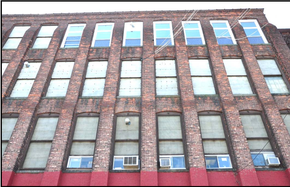
HALL 9: detail view of 1899 building, looking S from Fulton St., showing vinyl window replacements made to accommodate tenant reuse.
