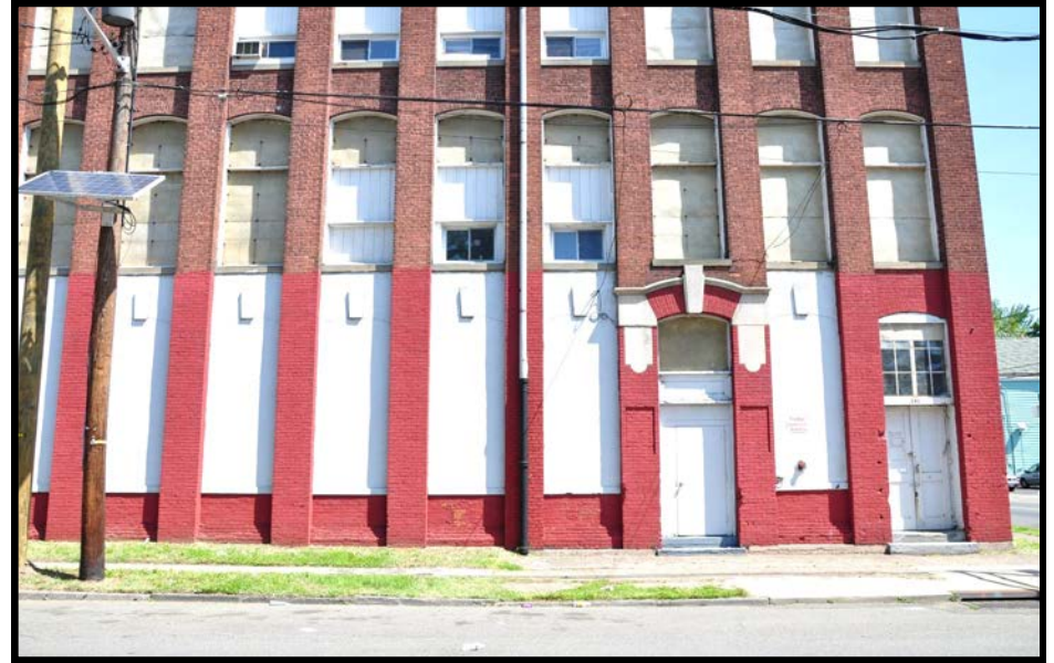
ARONSOHN 10: Detail view of west entrance on North side. Note the semi segmental hooded pediment with exaggerated keystone, which are classicizing elements that are indicative of F.W. Wentworth's design of the building.
