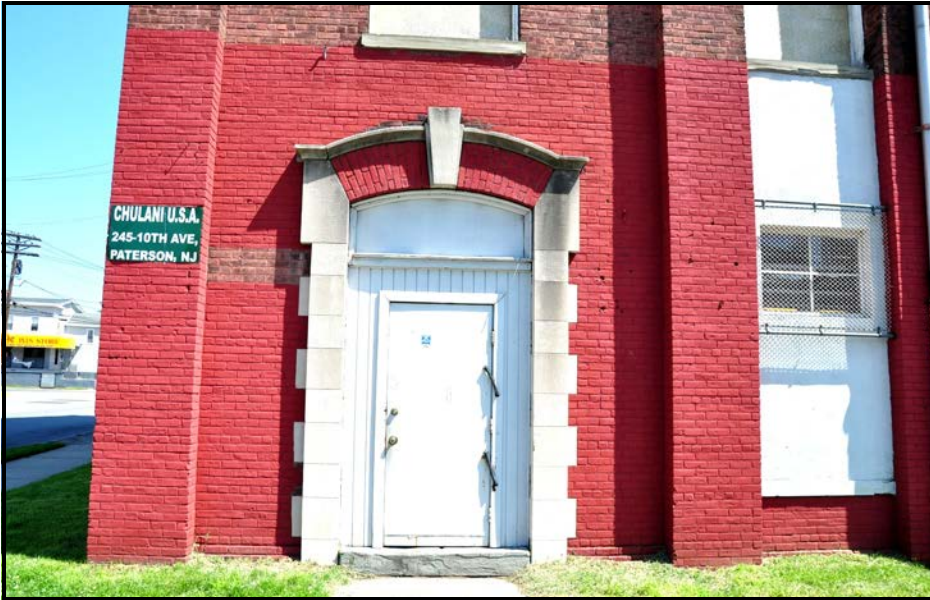
ARONSOHN 9: Detail view of east entrance on North side. Note the quioning and semi segmental hooded pediment with exaggerated keystone, which are classicizing elements that are indicative of F.W. Wentworth's design of the building.
