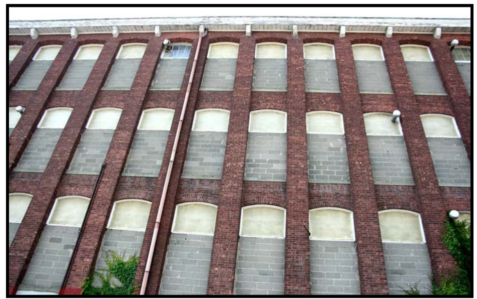
ARONSOHN 4: Detail view looking S from Tenth Ave. sidewalk. Note double hung window frames are intact, but lights have been replaced consistently with concrete block infill.
