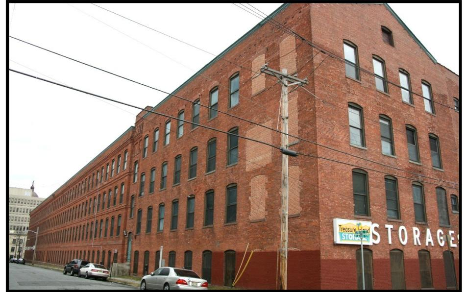
**BABOUR 14:** oblique view looking NE, showing Spring St. side. The joint between the 1877 building and the 1890 building is evident at left of center.
