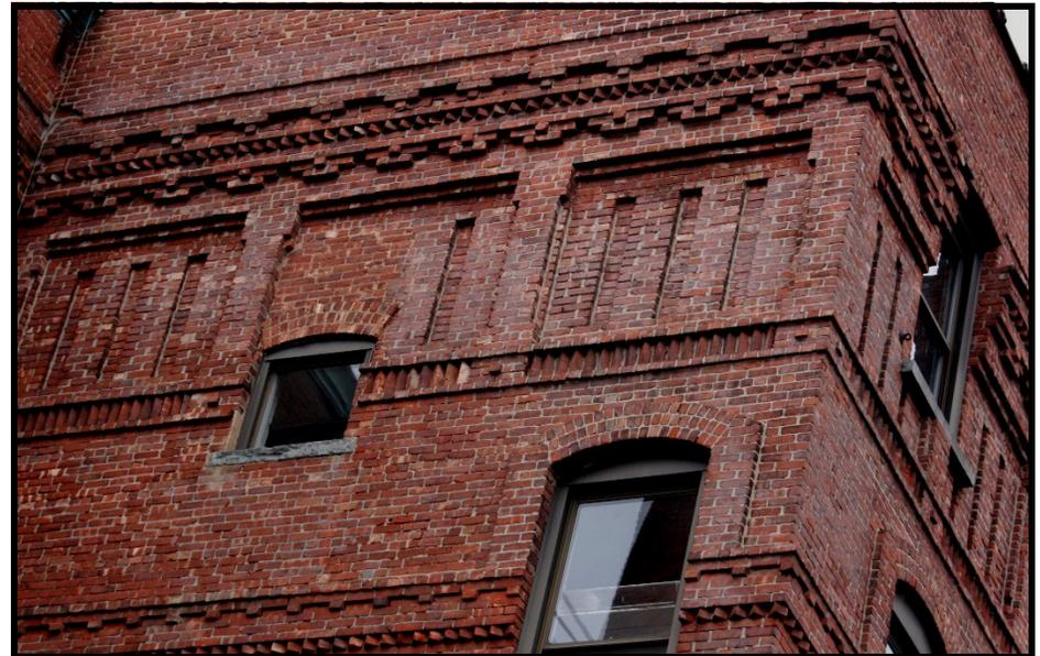
**BABOUR 12:** close up view looking NW from interior courtyard. Note the extensive brick detail and corbelling in this view of the 1877 original building.
