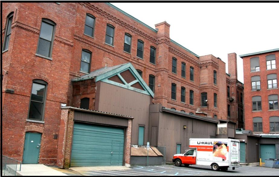
**BABOUR 11:** oblique view looking NW into 1877 building. The rolling door and trestle area at center mark the location of the Boiler House that has been removed.
