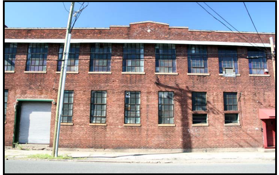
INTERNATIONAL 2: view of south façade of east building, looking north from across First Ave. Note steel sash windows remain authentic and intact overall.
