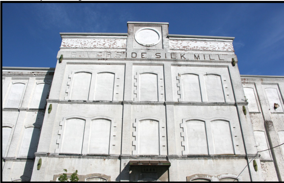
RIVER 3: detail view of central entrance bay of S façade looking N from River St. classicizing embellishments are present, such as the cast stone surrounds and quoining effects on windows, central oculus, faux pilaster columns, and string courses.
