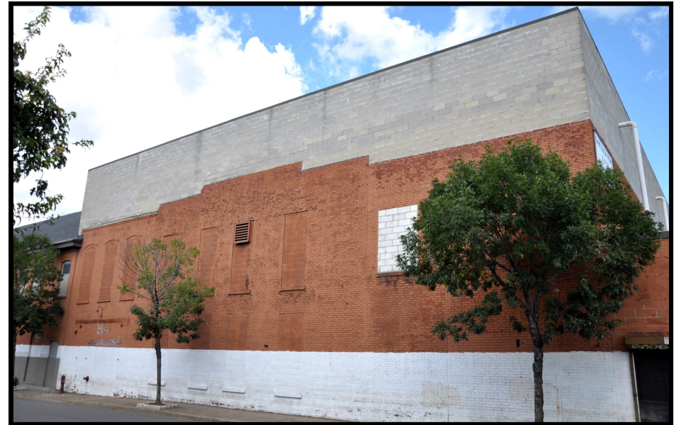
THONNERIEUX 6: view of south side of the eastern-most Dye House, looking north from 6th Ave. Note recent concrete block addition to the roof line.
