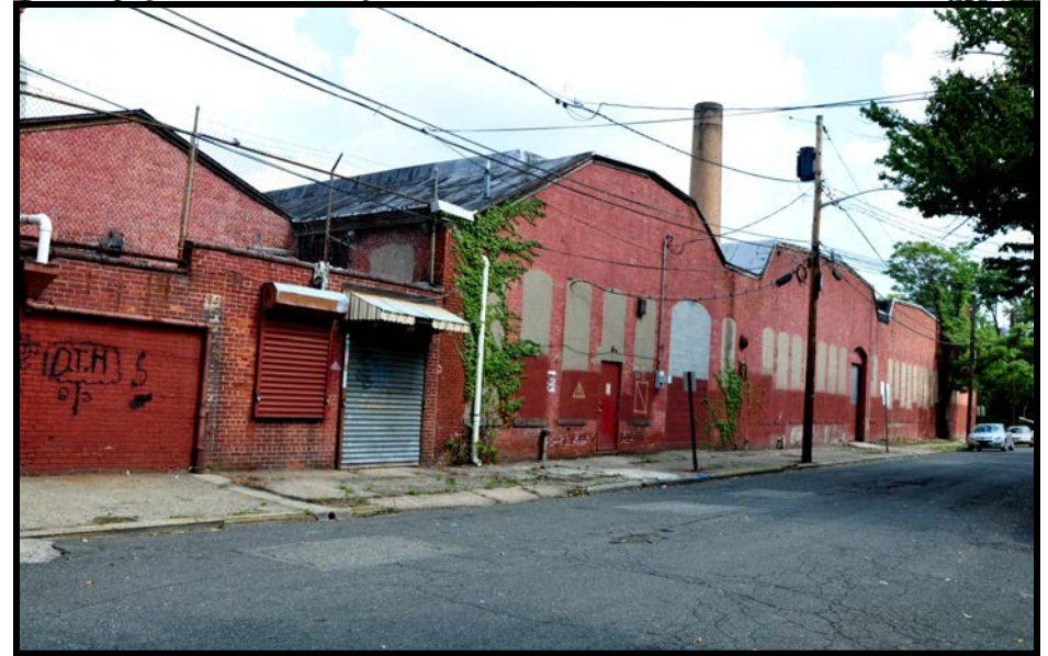
NATIONAL 4: oblique overview of Dye / Weighing Houses, looking southeast along Piercy St from about mid point of the complex.
