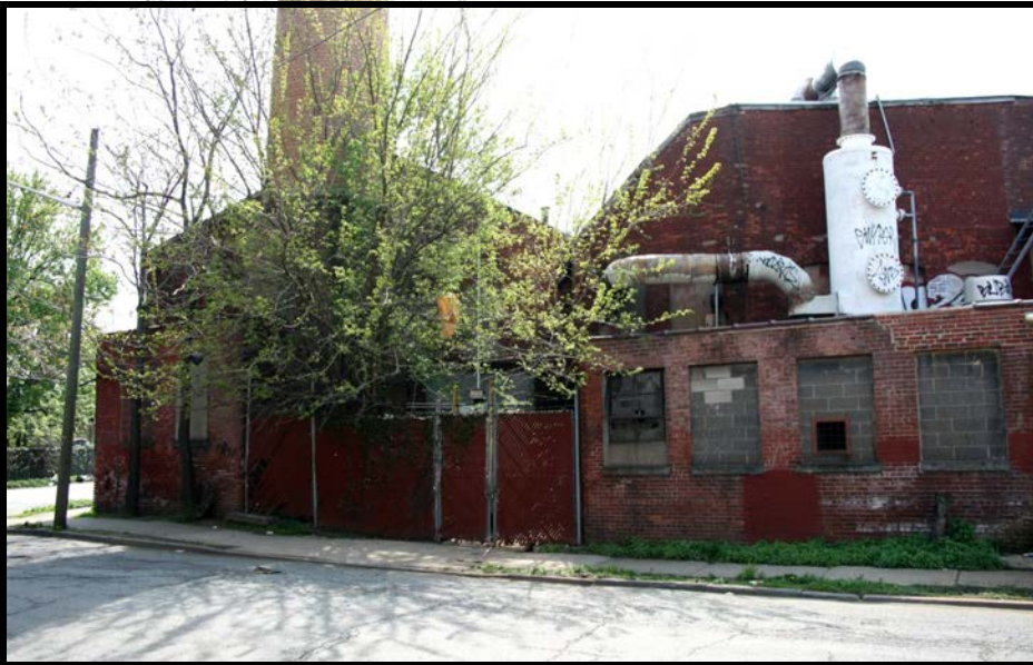
NATIONAL 7: Overview of north side of the complex, looking southwest from East Main St., Boiler House at left frame, and rear of Dye House at right frame.
