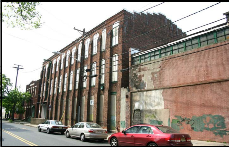
SIPP 5: Oblique overview of the Sipp Machine Shop, looking northwest from across Keen St. Features of note are its stepped pilasters, cornice corbelling, and stepped parapet. The Sipp Office Building is adjacent to the shop at right frame.
