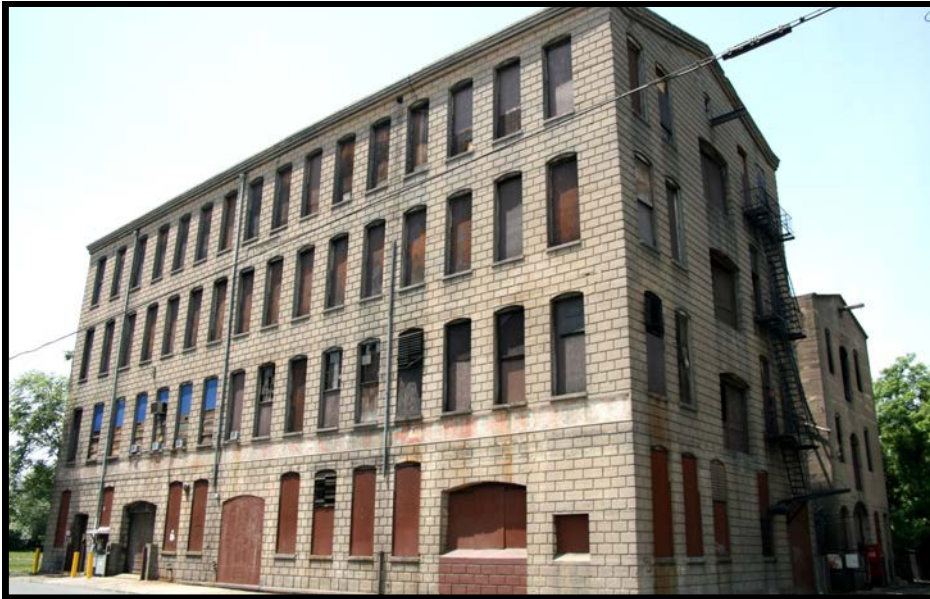
SOWERBUTT 1: oblique overview of west side of 1906 mill, looking southwest from across Paterson St. showing part of both gable ends and full west elevation.
