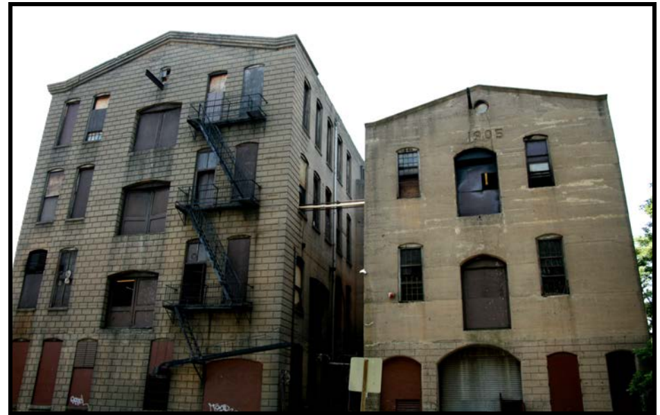
SOWERBUTT 4: oblique overview of north gable ends of both mills, looking south from Harrison St.
