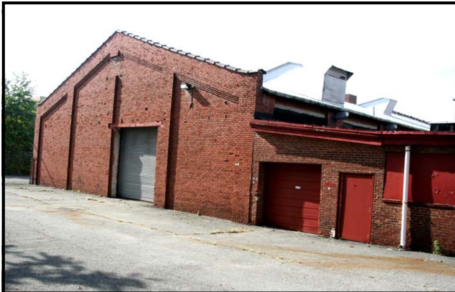
MIESCH 3: Silk Printing shop, oblique view looking NW showing S façade. Note intact cornice detail, and later addition of rolling door entrance and side wing infill.
