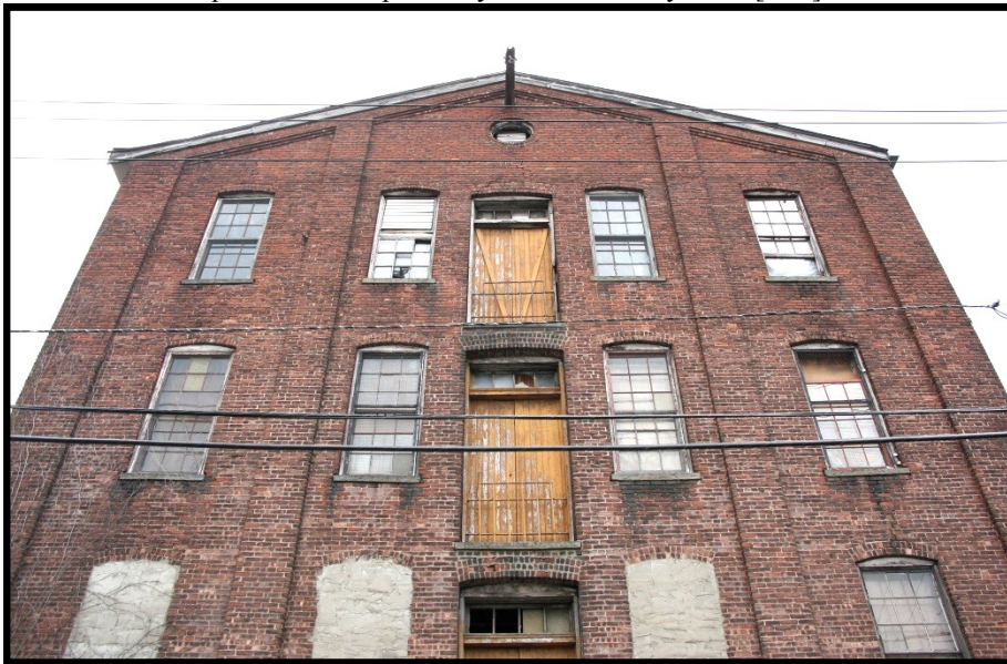
MIESCH 3: Detail of 1890 mill Courtland St. façade looking N. Note the number of intact double hung windows, central loading doors, central oculus window, stepped corbel detailing and pilaster articulation as character defining features.
