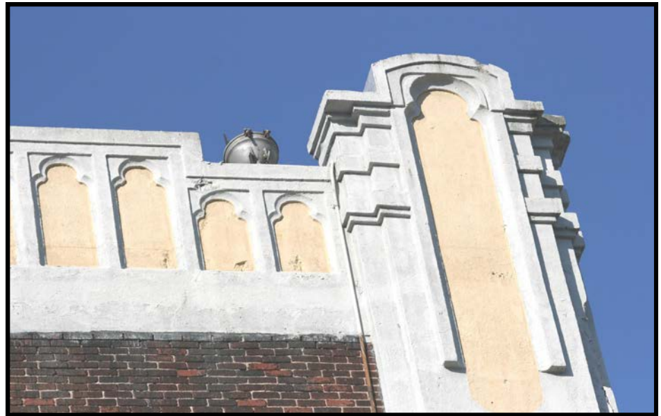
WRIGHT 6: close up view of S end of Bld. 1, looking N, showing geometrical parapet detailing in cast concrete. Such detail sets Bld. 1 apart from the complex additions made after this first bld was designed by F.W. Wentworth in 1915.
