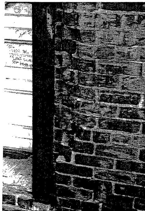
Typical damage to brick at a loading door, where it has not been protected by a steel bollard or angle.
