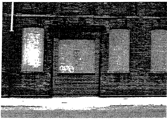
Note the historic steel door frame that was left in place when this loading door was bricked in.
