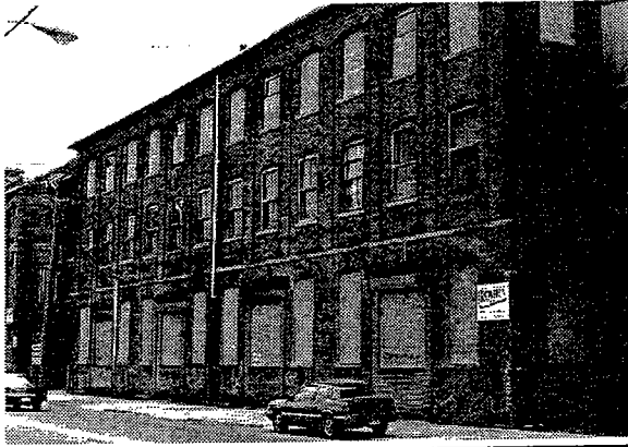
The window openings at the Rogers Locomotive Frame Fitting Shop were bricked up in a manner that leaves the original openings discernible, but has altered the appearance and character of the building.
