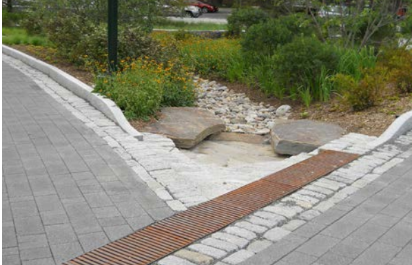
Vegetated Stormwater Inlet, Philadelphia PA
