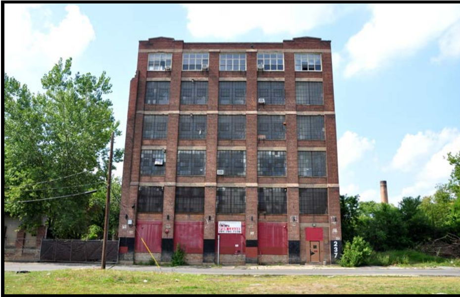
MANHATTAN 1: overview of south façade of the only remaining intact building of the complex, looking north from across River St. Note steel sash windows intact.
