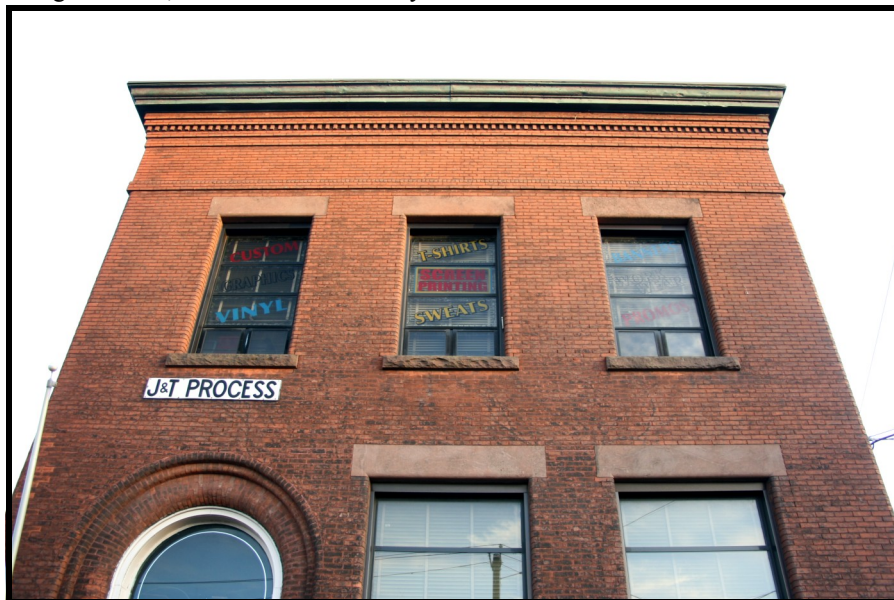
COOKE 3: Administration Building, looking S, showing N façade. Note intact cornice detail, dentils, sandstone lintels, cut stone sills, rounded brick circular entrance.
