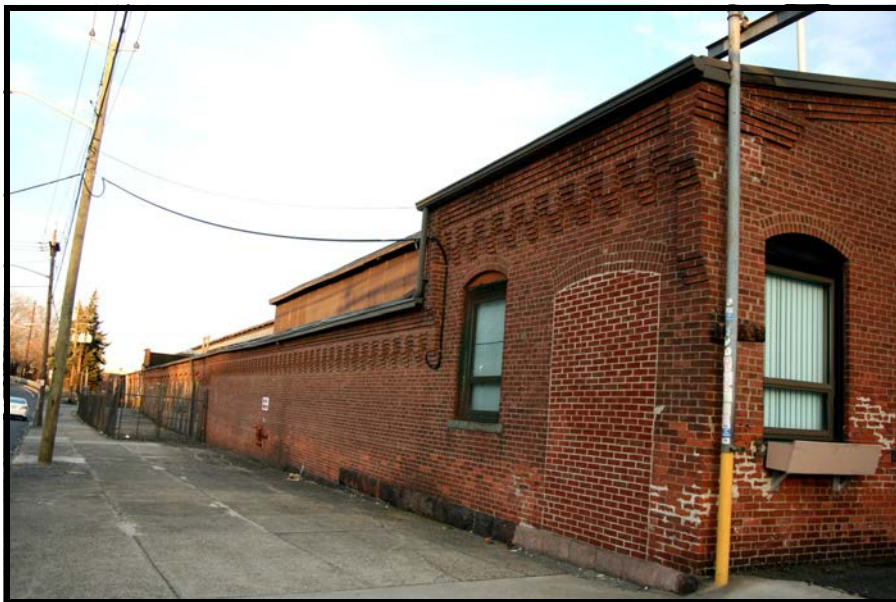
COOKE 7: Wash House & Machine Shop, looking SE, Madison Ave at left. Note intact corbelling detail running length of the 200 ft. machine shop.
