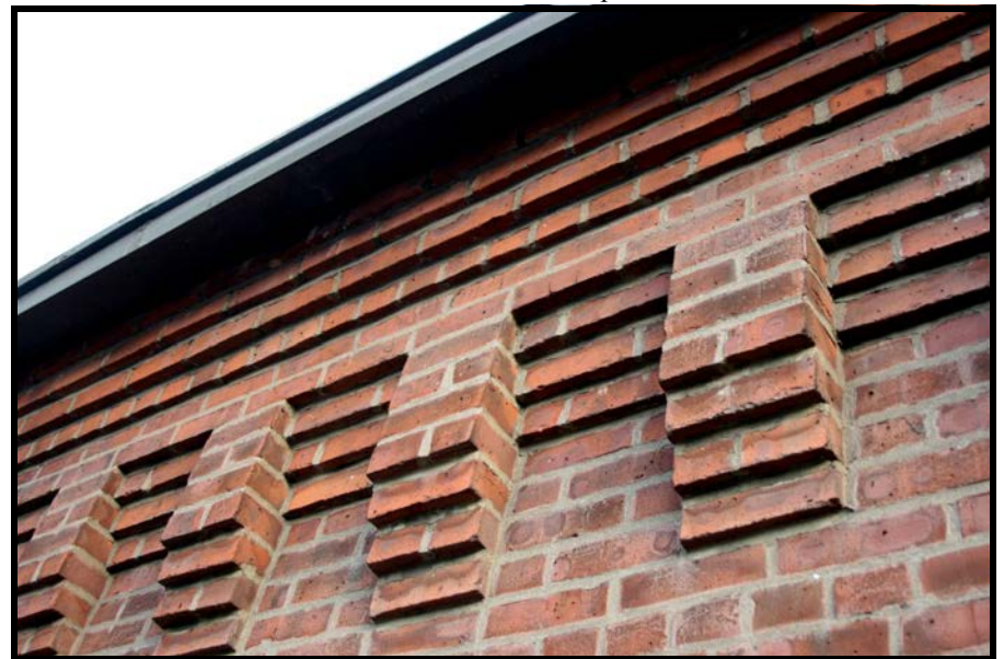
COOKE 8: detail view of stepped corbelling detail along cornice of Machine Shop.
