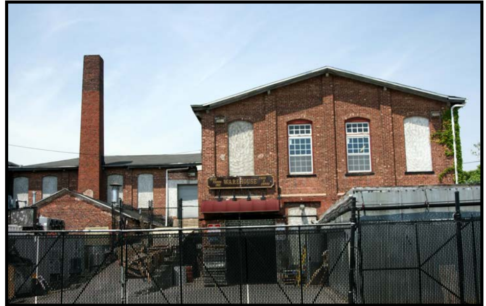
SAVOY 2: View looking west of the northern-most mill, showing its east gable end, and the boiler house and square smokestack to the left of frame.
